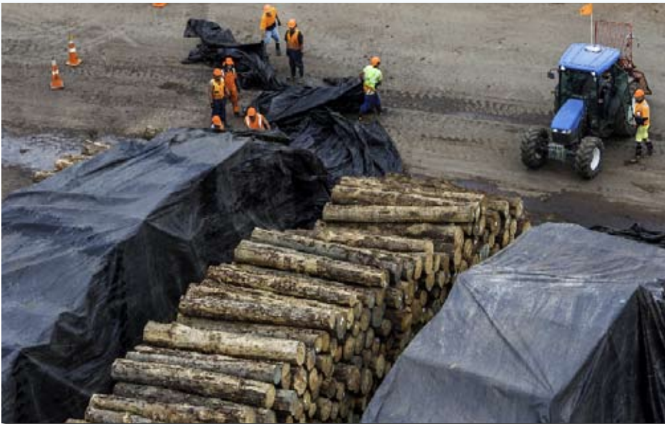
Placing Tarpaulins over log rows
